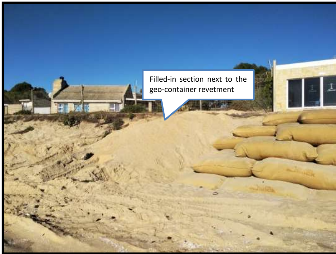
Figure 9: Filled in section next to the geo-container structure
