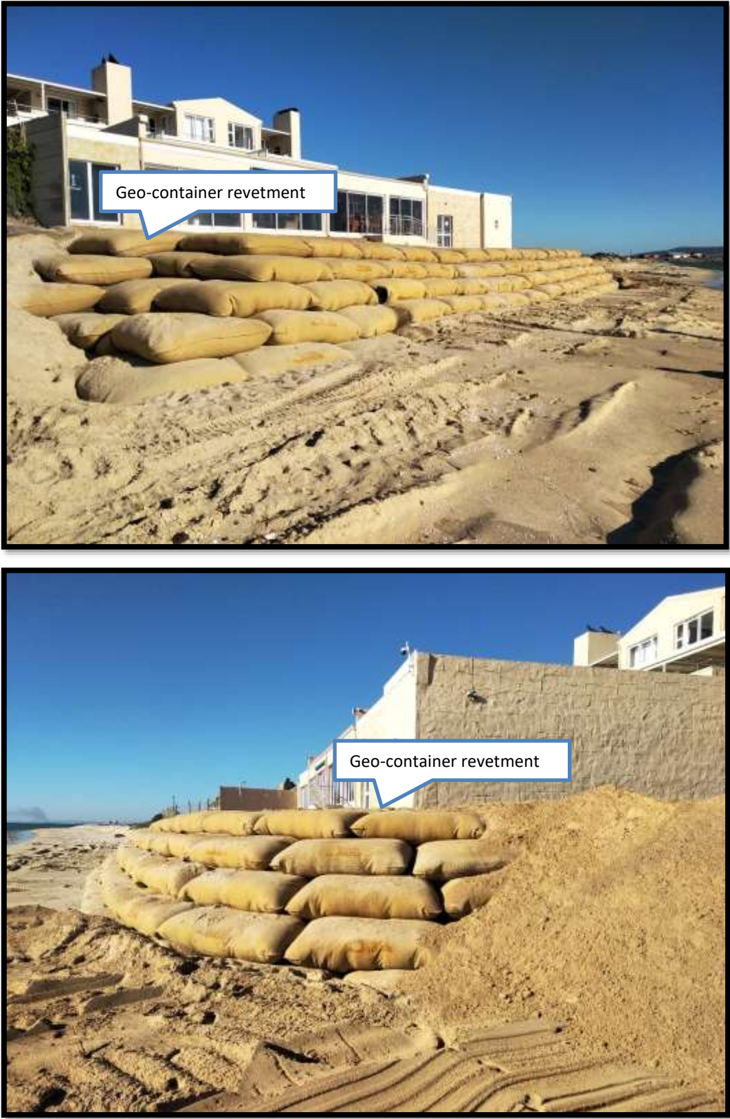
Figure 6: Completed geo-container structure
