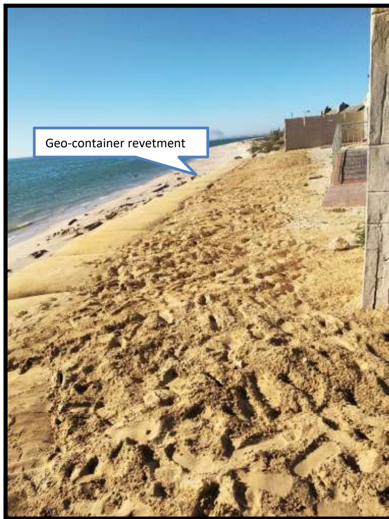
Figure 7: Top part of the geo-container structure
