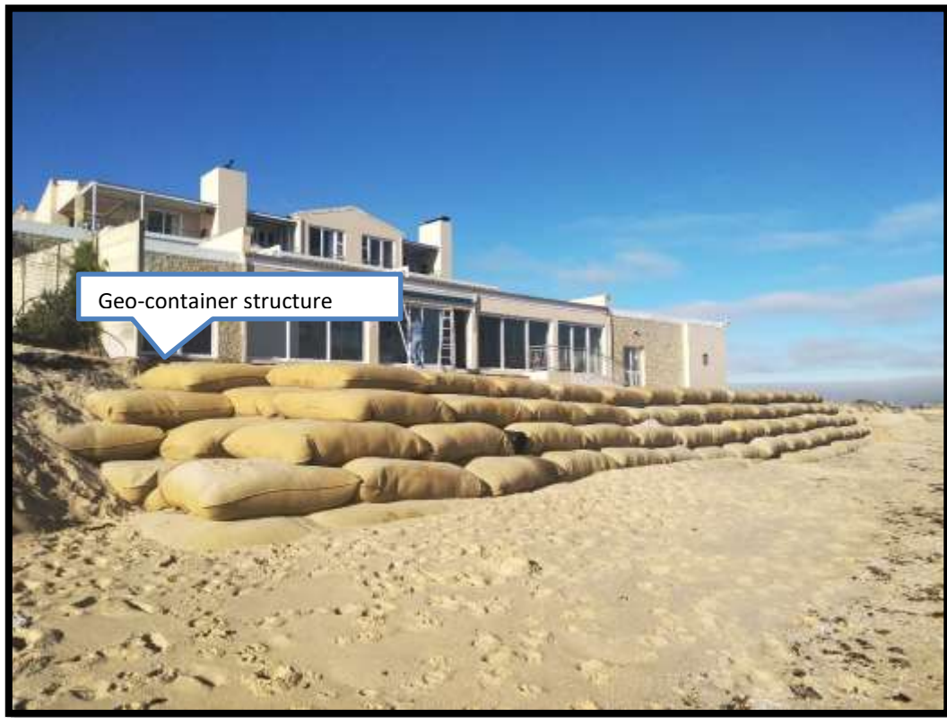
Figure 14: Completed geo-container structure
